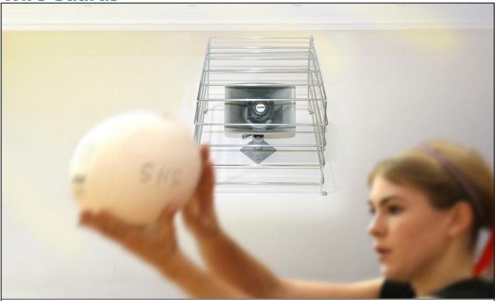
Valcom's Wire Guards provide an extra layer of protection for horns and speakers in high damage areas such as school yards, gymnasiums, prisons and manufacturing facilities where vandalism and accidental damage can occur. The wire guard is designed of heavy gauge construction and is zinc plated to help prevent corrosion from environmental elements.
